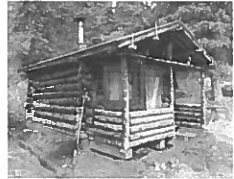
The Upper Toklat Patrol Cabin was preserved through rehabilitation
